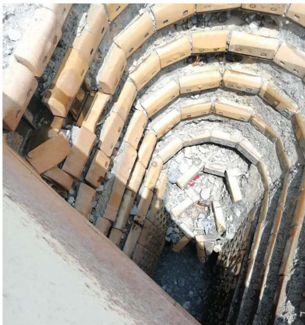
OPENING IN CHUTE PLATEWORK
